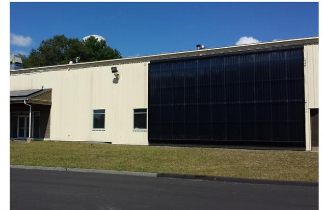
*This solar heat reduces the amount of fuel used for space heating.*
