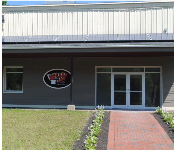
Clean energy efficiently powers the Wicked Joe coffee roasting facility in Topsham, Maine.
